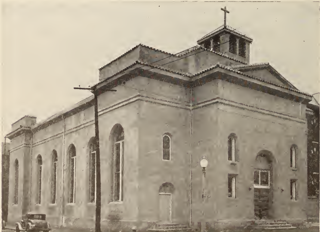
Old St. Patrick's Church after modernization with Portland Cement Stucco over metal lath
